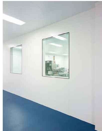
GMP wallsystem with cutouts for windows
